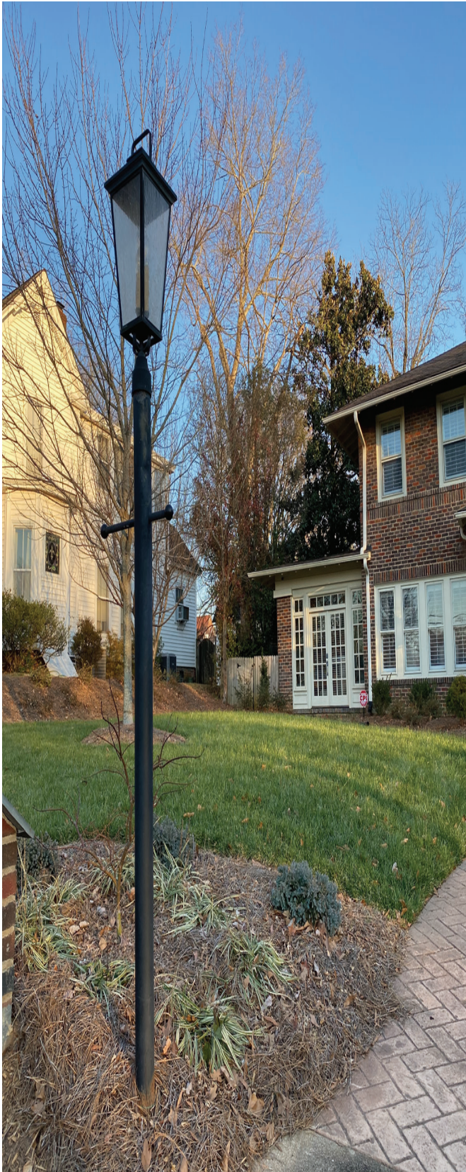
EXISTING POST & ELECTRIC LIGHT
